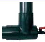
Installation of valves and cocks for sampling and draining.
